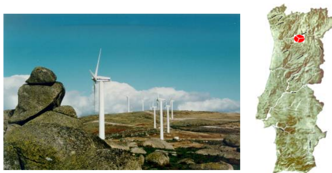
Figure 1 – Fonte da Mesa Wind farm
